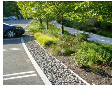
Image 17 Pervious, landscaped surfaces and light reflective surfaces minimize heat absorption.
